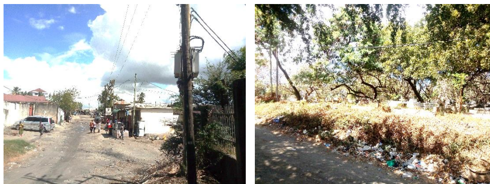
Figure 4: Power lines and Cemetery at Mivinjeni street
